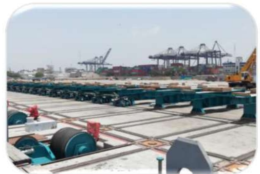
Fabrication of SLTS Platform
