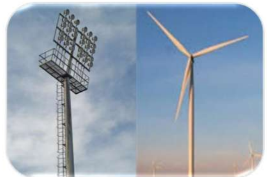
Flood Light & Wind Turbine Towers
